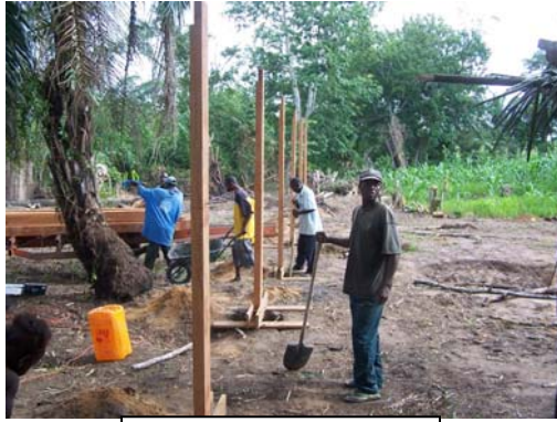
Columns being set
