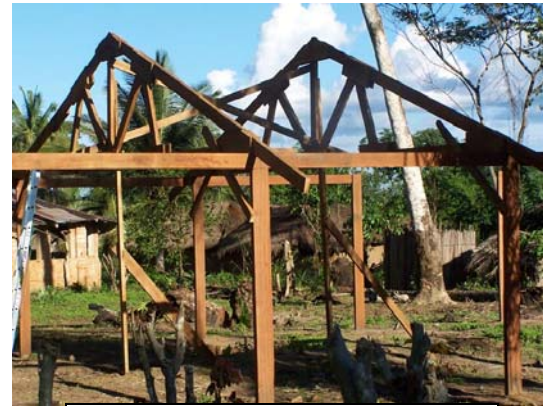
Trusses in place and braced
