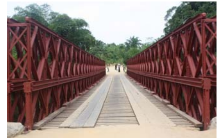
The Lokenye bridge rebuilt
